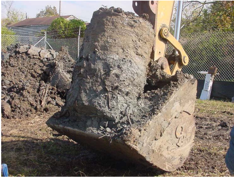
Photograph 1. Excavated test column.
