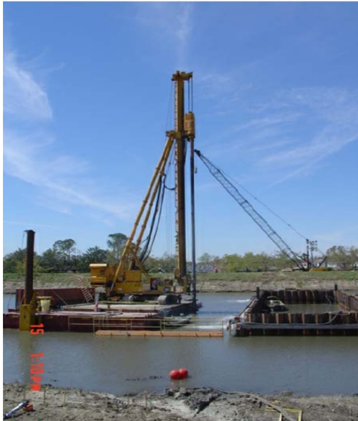
Photograph 3. DMM operations from barge at Orleans Avenue Canal, New Orleans.
